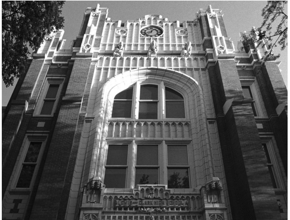
Dedicated in 1912, the Lewis & Clark High School in Spokane, Wash., was renovated and expanded, preserving the building's architectural grandeur while modernizing the facility for some 3 percent less than new construction would have cost.
